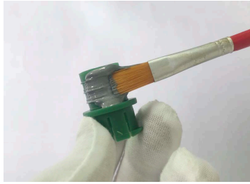
Apply cement on socket
