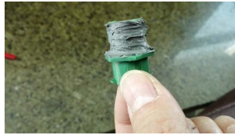
Socket with cement layer
