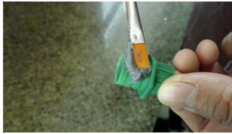
Apply cement on socket
