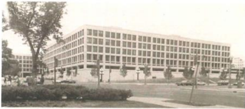
UNDER GSA MANAGEMENT , the new U.S. Department of Labor Building and the new U.S. Tax Court Building are both cooled by centrifugal machines that are "cleaning up" on energy savings.
